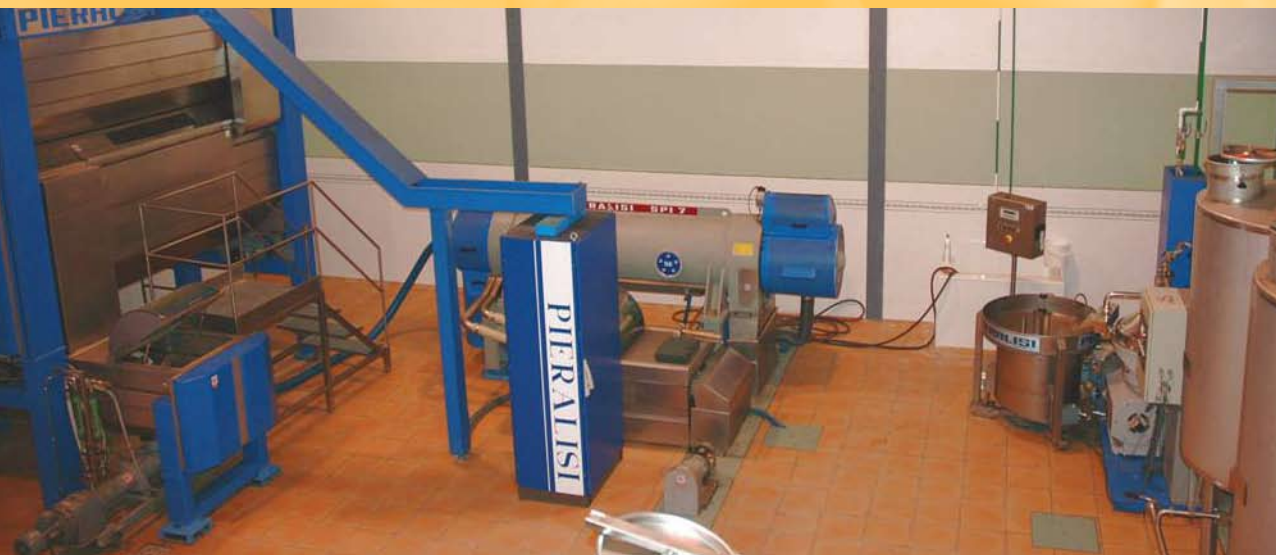
Two-step Extraction System at the Montilla Mill
